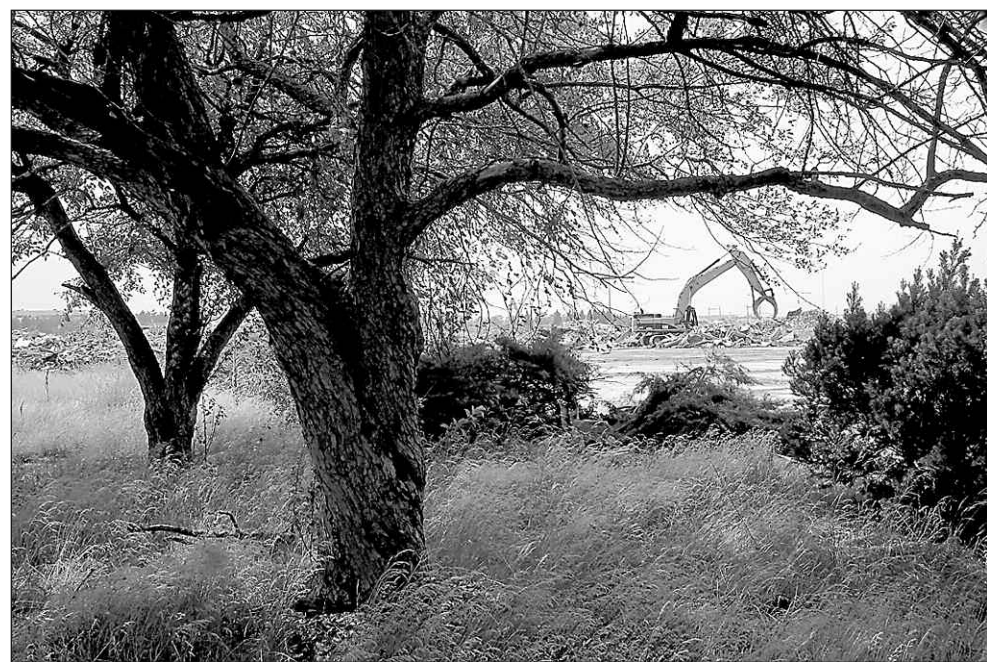
A trackhoe takes prey Tuesday on what used to be, the truck plant at Opdyke and South Blvd.
